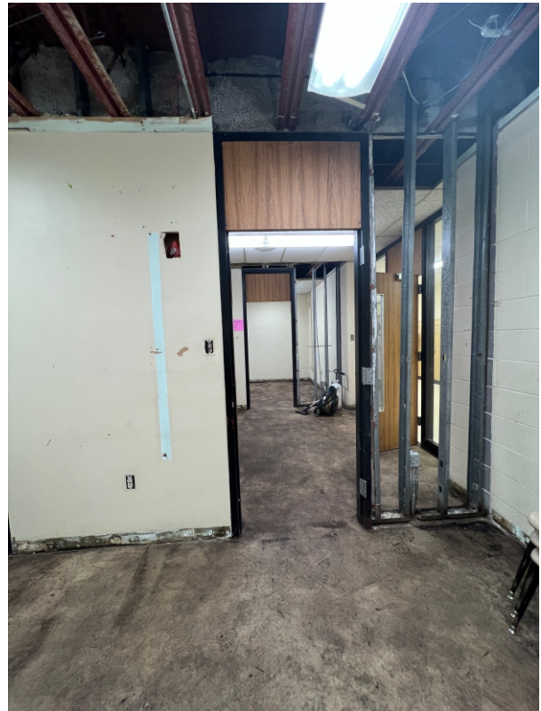
Westropp probable ACM on conc.
